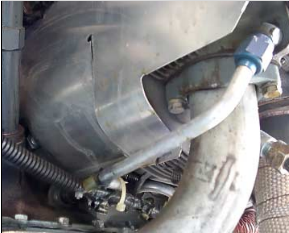
Detail view of the bottom of the rear right (RR) baffle (installed), view from the bottom.
