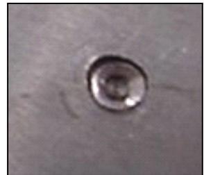
To replace a rivet, first drill off the head; then push the rest of the rivet through.
