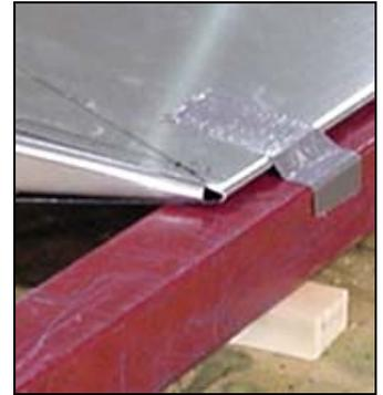
Remember always have the 3/4" spacer block under bottom trailing edge.
