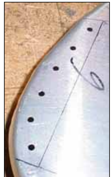
Rivet pattern and slat support trace line.
