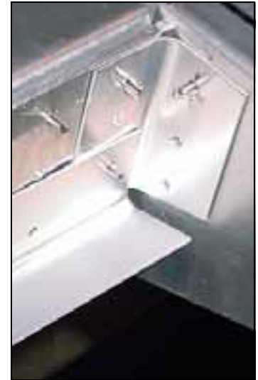
L angle overlaps corner L angle.
