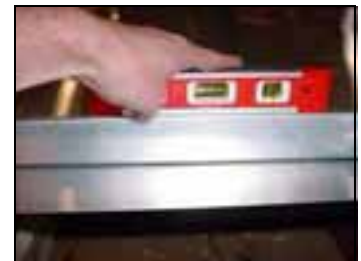
Between the ribs, check that the rear channels are level.
