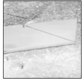
Layout the diagonal cut line on the vertical flange.
