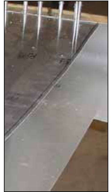
Rough cut the sink approximately 10mm oversized.
