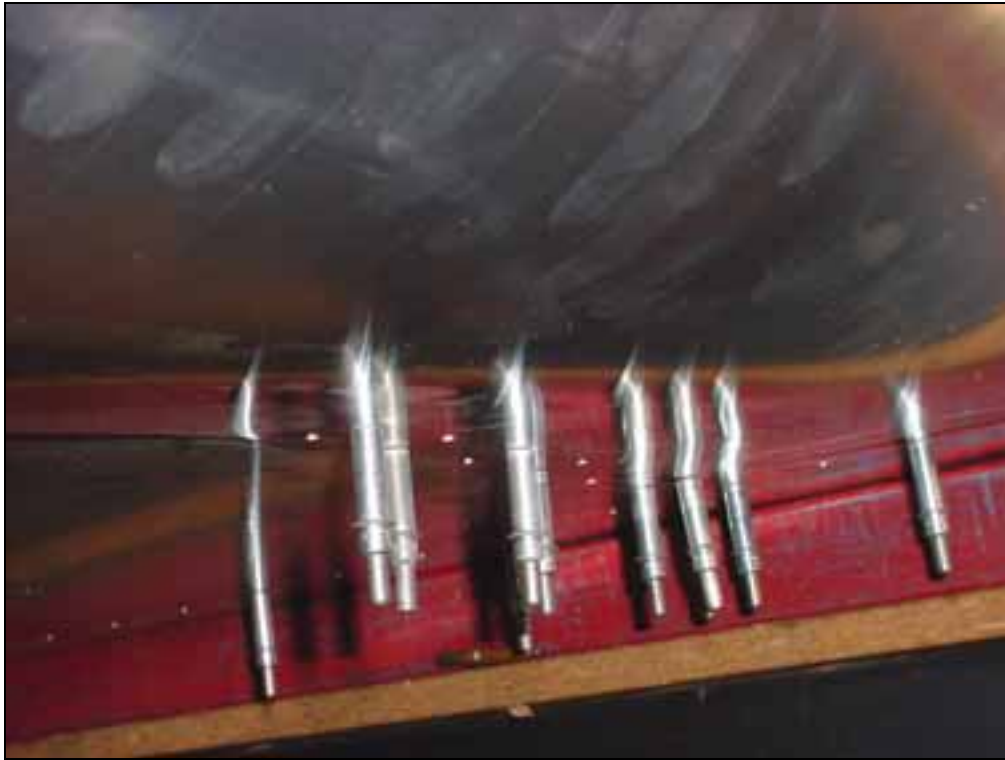
Drill and Cleco the bottom side.
