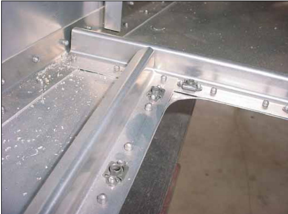
Rear right detail. Z angle overlap on top of the Longeron 6B2-1 Flanges overlap up to the bend tangent line.
