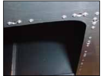
Looking up and forward, rear right corner.
