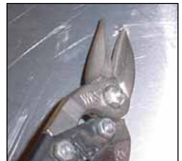
Cut out the opening.
