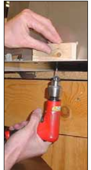
Wood backing block on top side.
