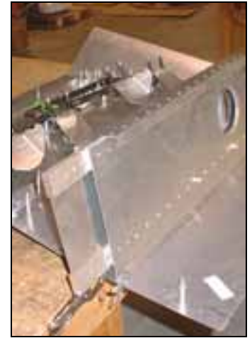
CHECK: Spar rivet line is visible through the pre-drilled holes in the cabin floor skin.
