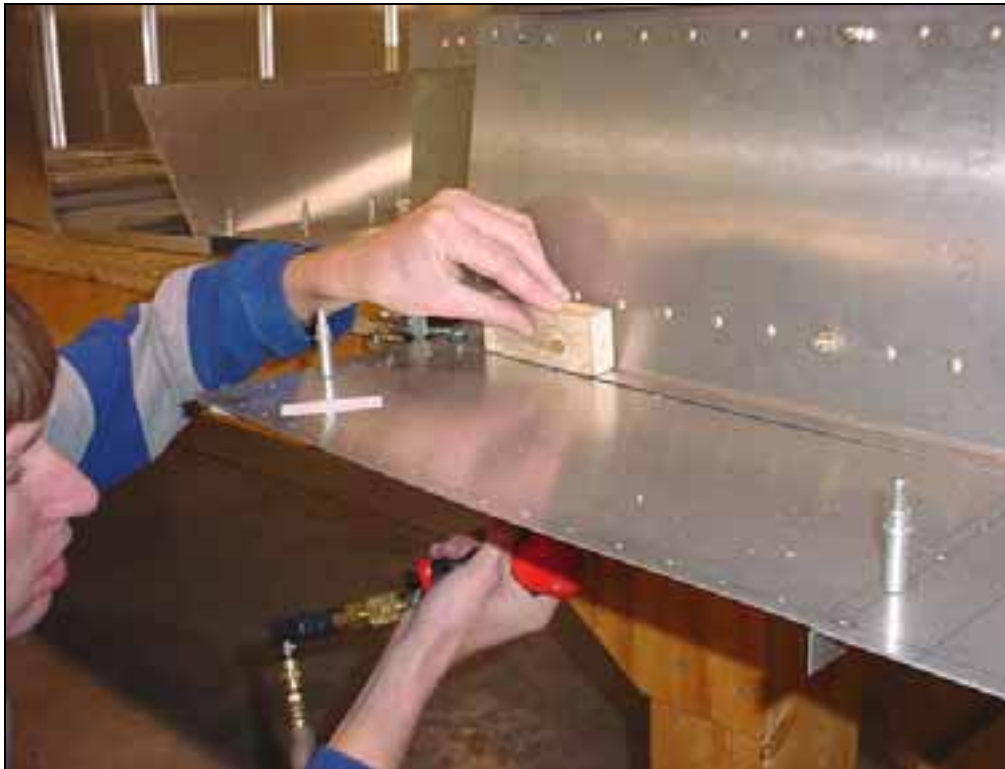
Back drill and cleco.
