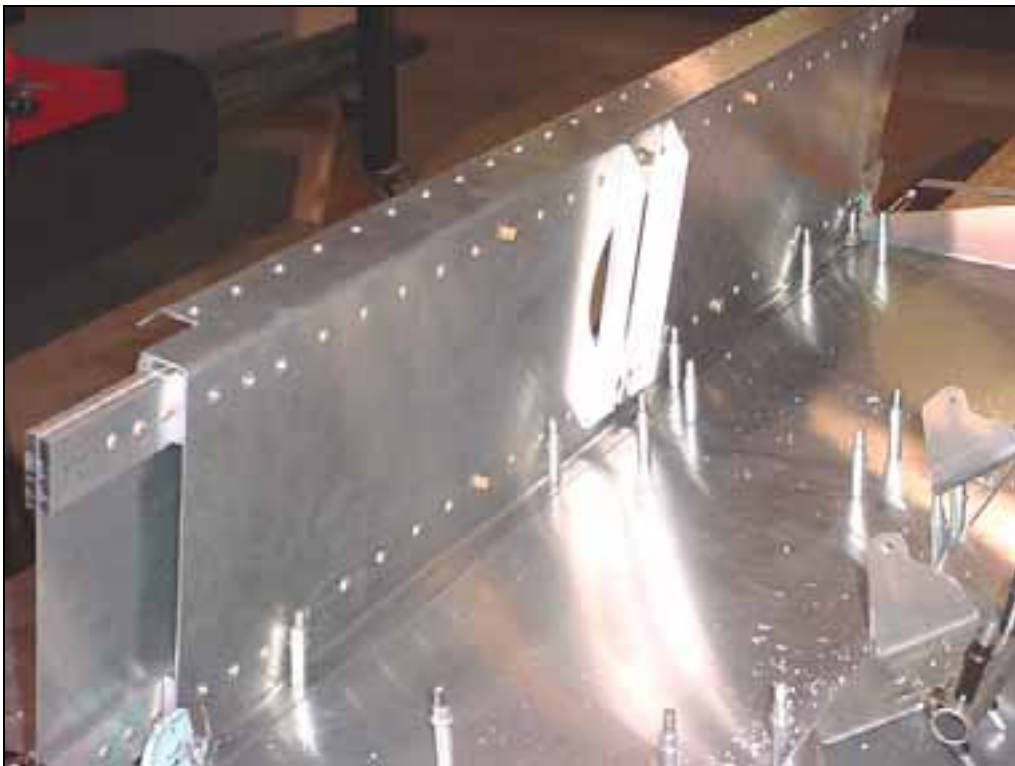
Aft side of spar. Finish drilling the rivet line.
