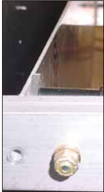
The top of the web must be flush with the top of the spar insert.
