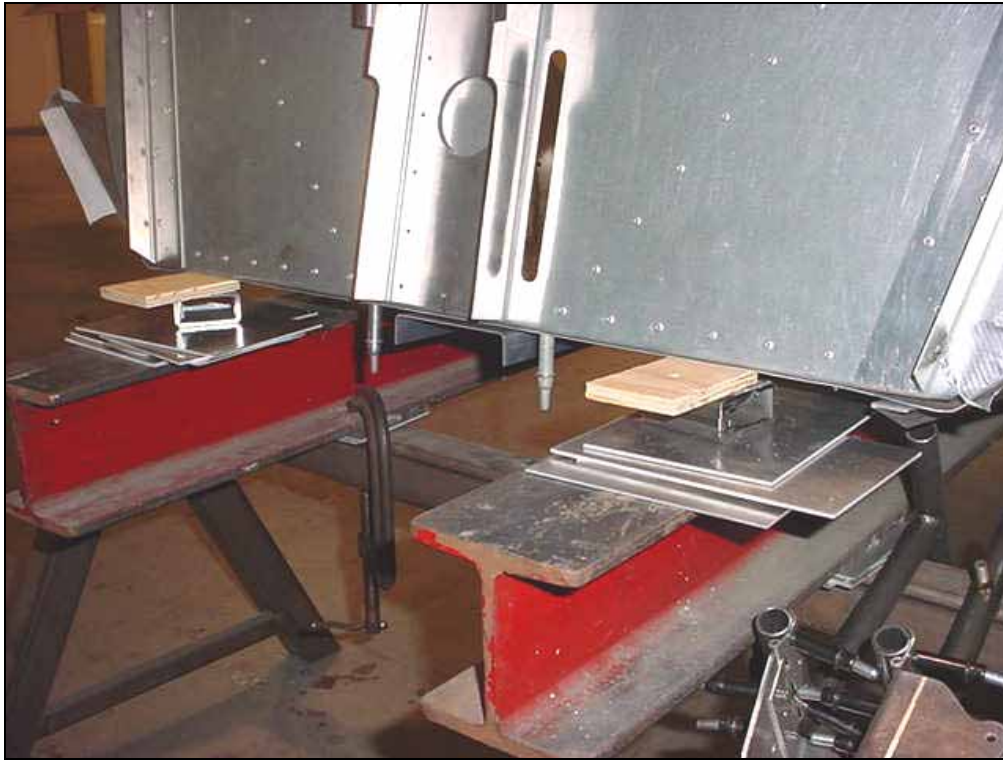
Detail of the spacers underneath the front edge of the cabin floor.
