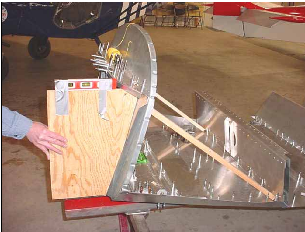
Re-check the angle of the firewall, and plumb line.
