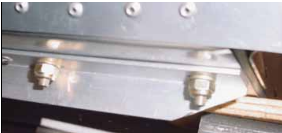
CHECK: The bolts are centered on the lower front longeron 6B10-3
