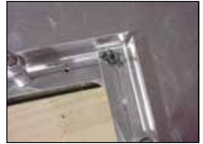
Before riveting the nutplate, drill the middle hole for the screw to \frac{1}{4} "
