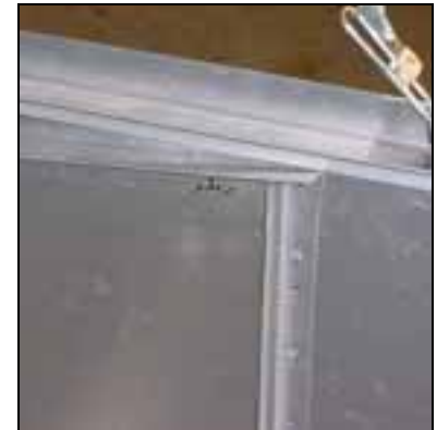
End of diagonal L angle even with aft edge of vertical L angle.
