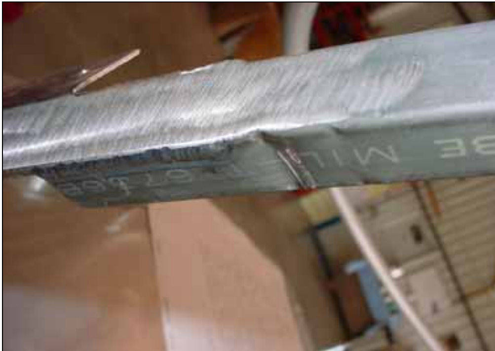
Photo of front underside of the canopy frame.
