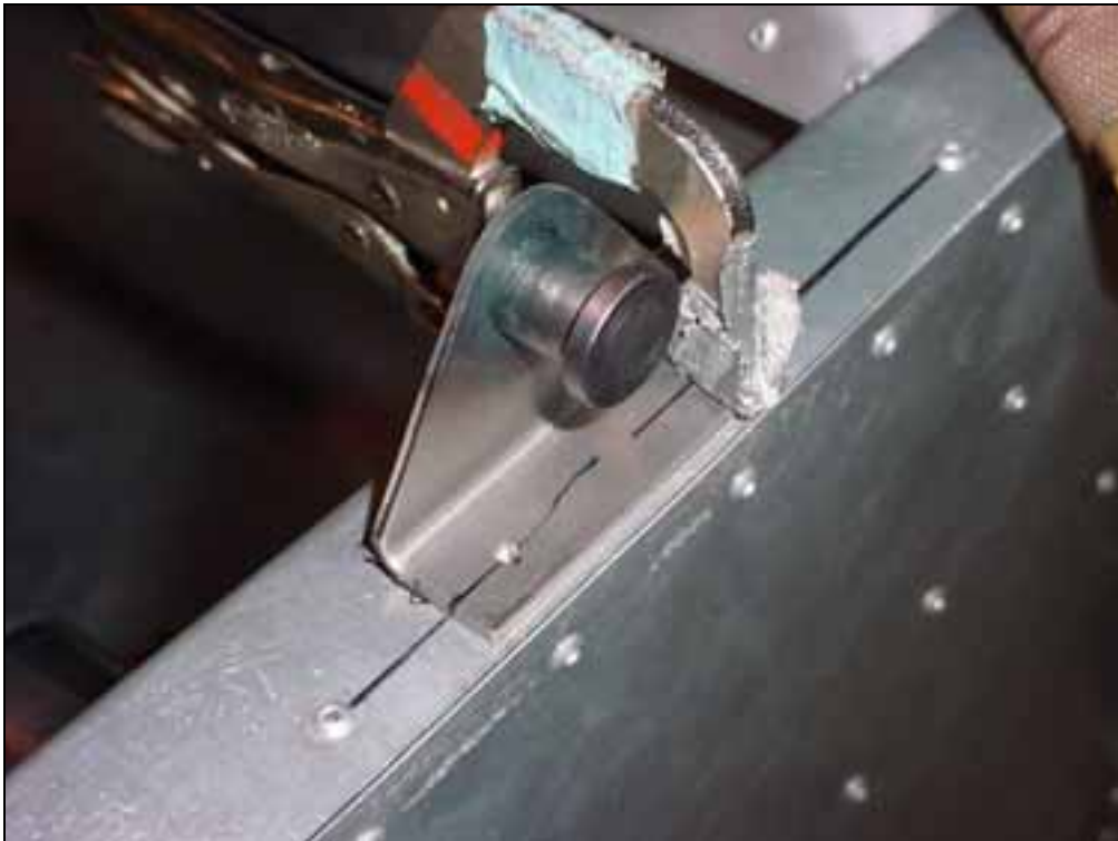
Mark the longeron center line on the bottom flange of the stud, Drill and Cleco.
