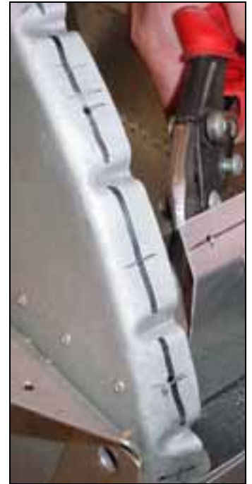
Use the snips to cut corner of flange.
