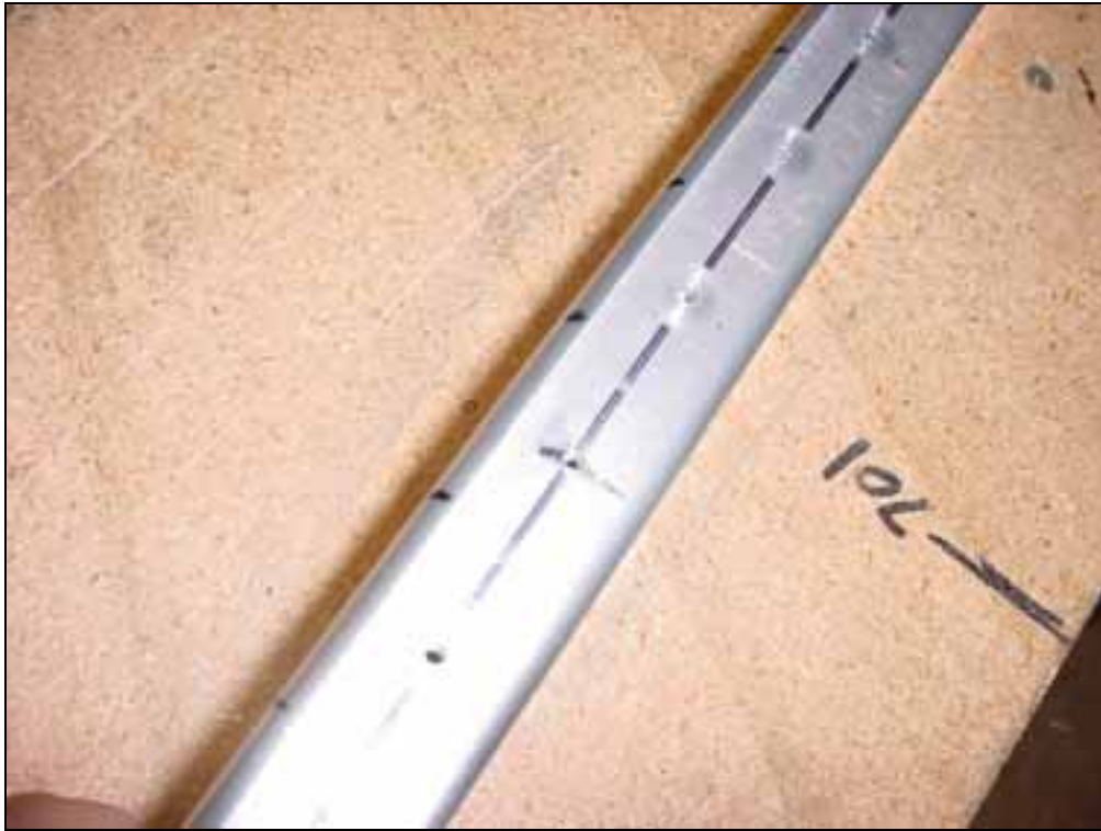
Top rivet line between the crimps.
