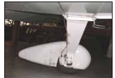
LEFT WHEEL. Above photo shows gear installed opposite of the recommended direction.
