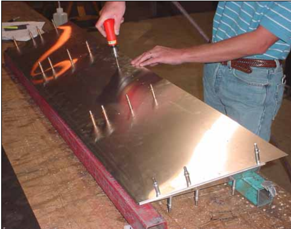
Turn the aileron over. Reposition the spacer block under the outboard trailing edge. Start in the middle, drill and cleco the front rivet line.
