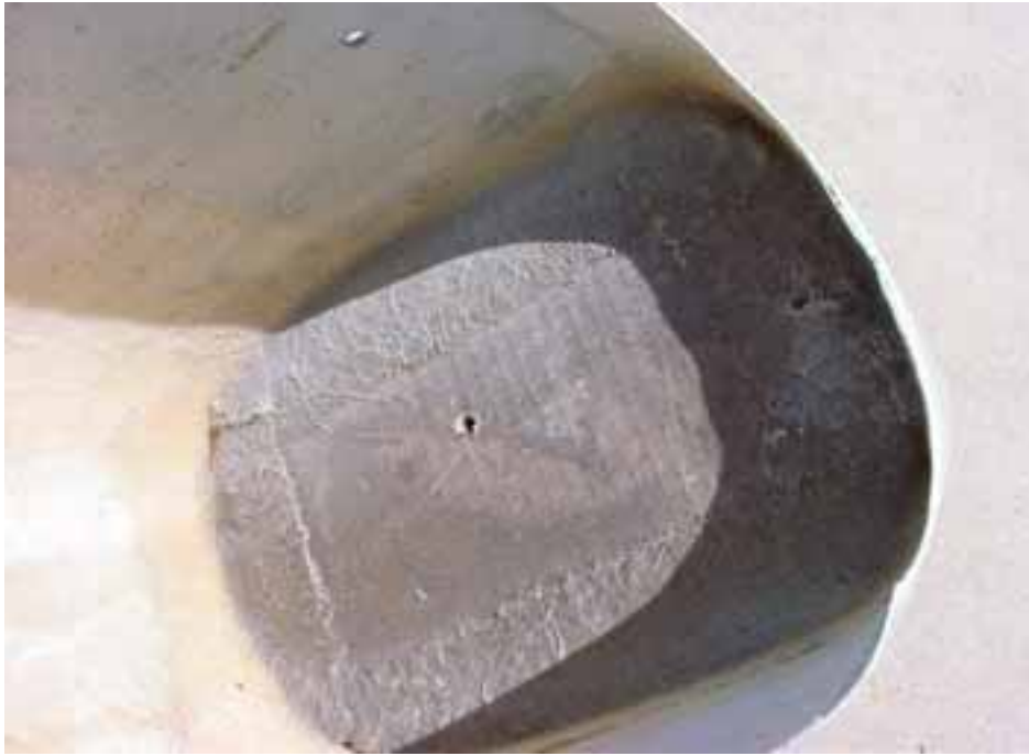
1/4" hole in bulkhead.
